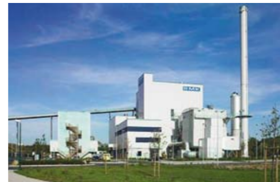
Biomass power plant Lünen, completely equipped with REITZ variable speed controlled primary air fans, secondary air fans, exhaust air re-circulation fans and ID fans. Photo: REMONDIS, Lünen
