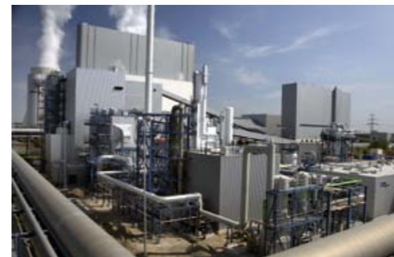
Oxyfuel pilot project Schwarze Pumpe by Vattenfall. Equipped with REITZ fans, the world's first CO 2 -free lignite-fired power plant is coming into existence. Photo: Vattenfall, Berlin
