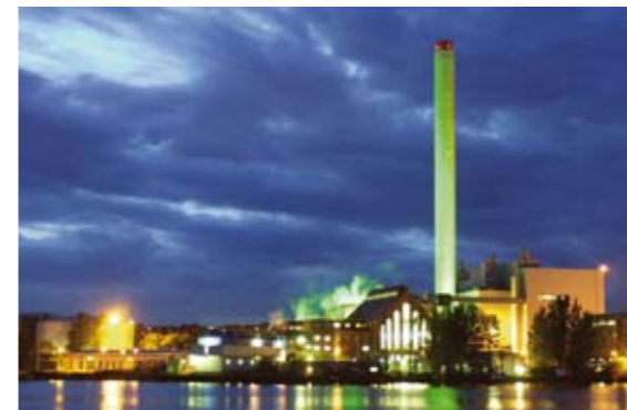
Power plant Flensburg, equipped with REITZ fans Photo: Stadtwerke Flensburg
