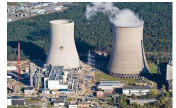
Natural gas power plant Lingen, equipped with REITZ fans. Photo: RWE Power
